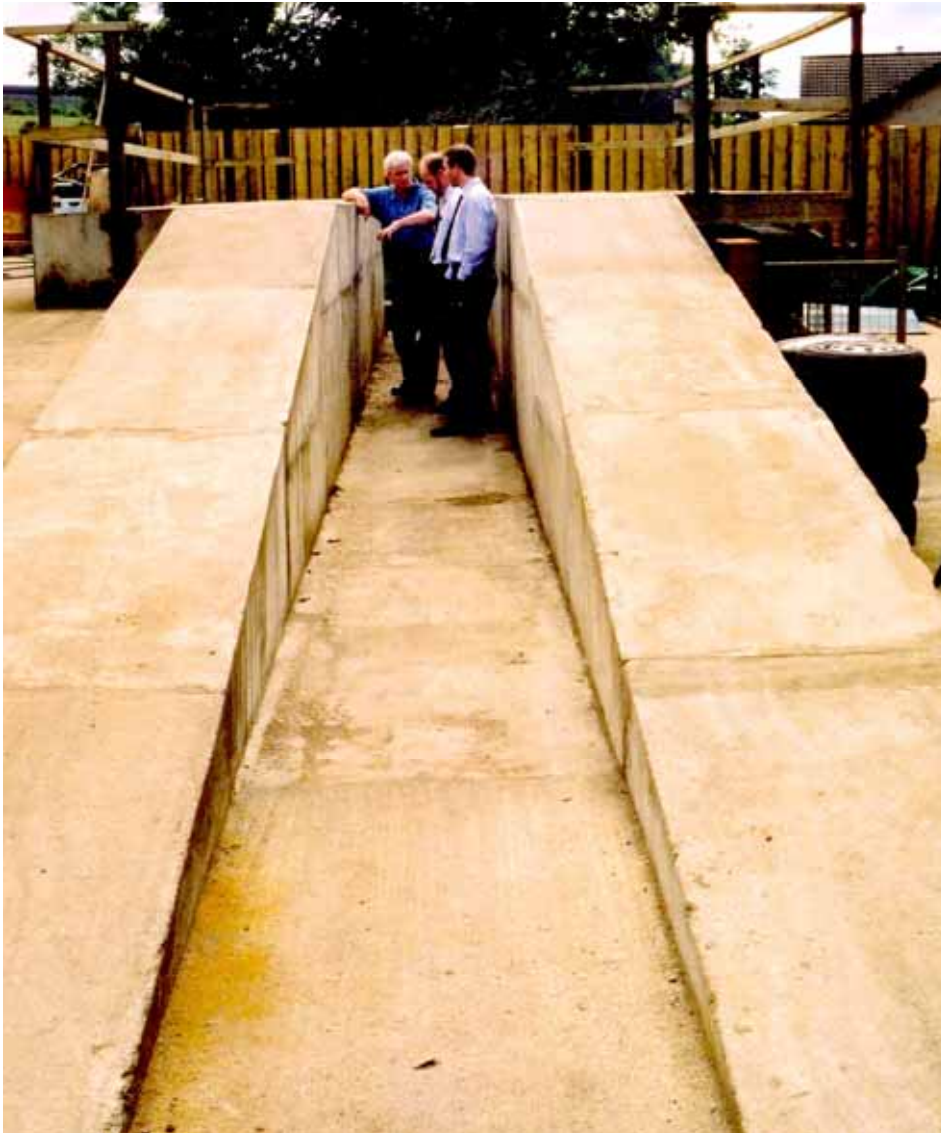
Figure 5.42 Car ramp constructed of tyre bale/concrete blocks (courtesy of TRL Ltd ©)
