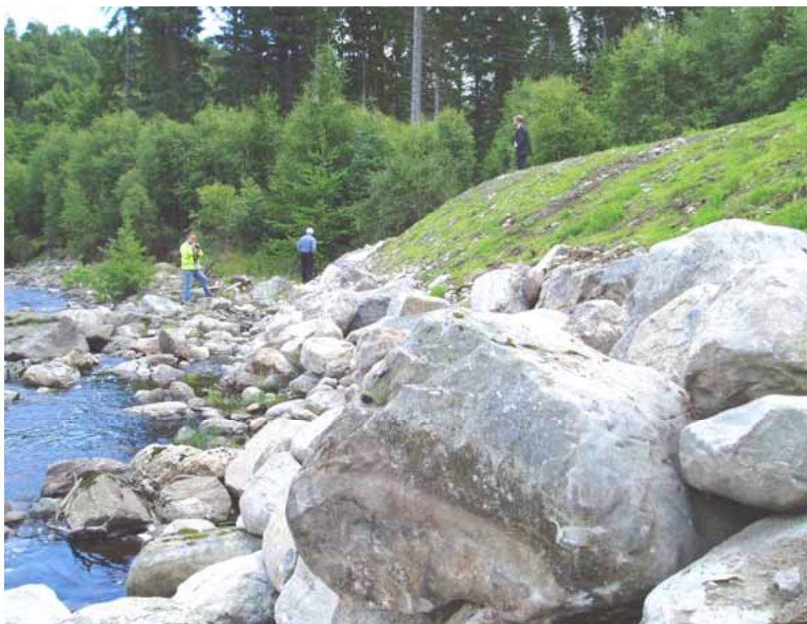
Figure 5.35 Rock armour placed for bank toe protection
