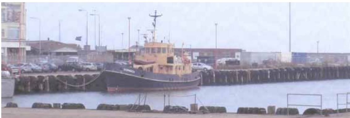
Figure 5.22 Tyres used as mooring fenders on Lowestoft wharf s (courtesy Sorrell Flood Protection)
