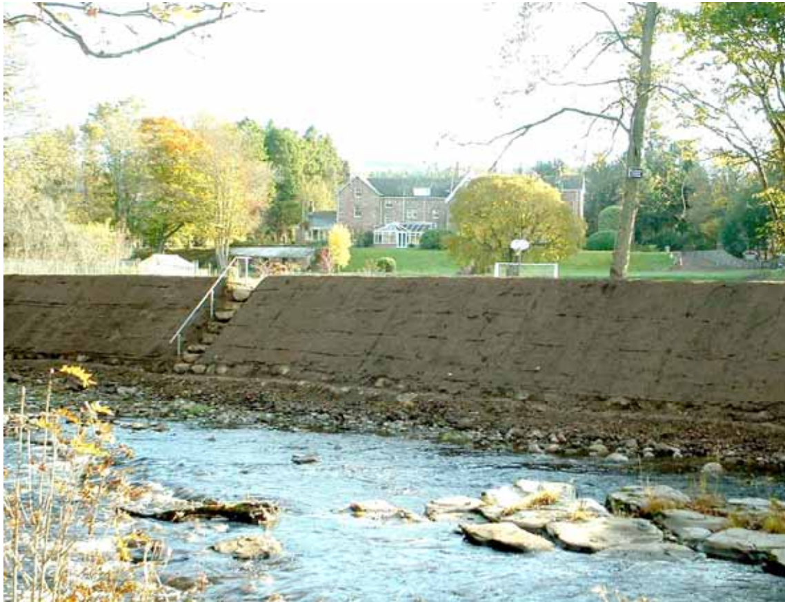
Figure 5.37 The Nairn river bank with topsoil replaced (courtesy Northern Tyre Recycling)
