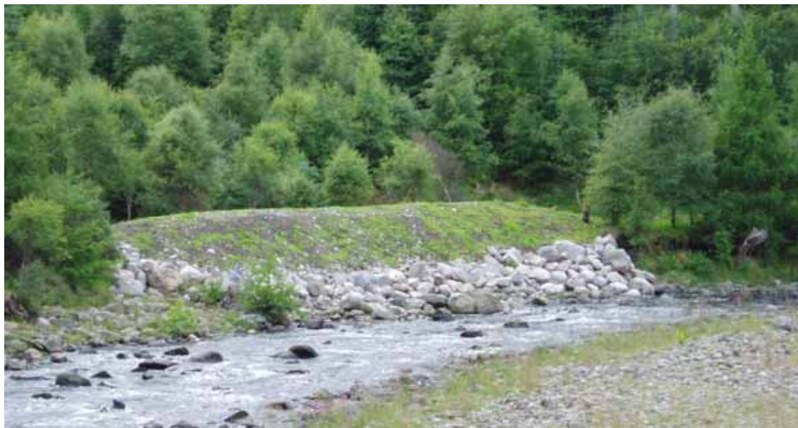
Figure 5.34 The finished river embankment
