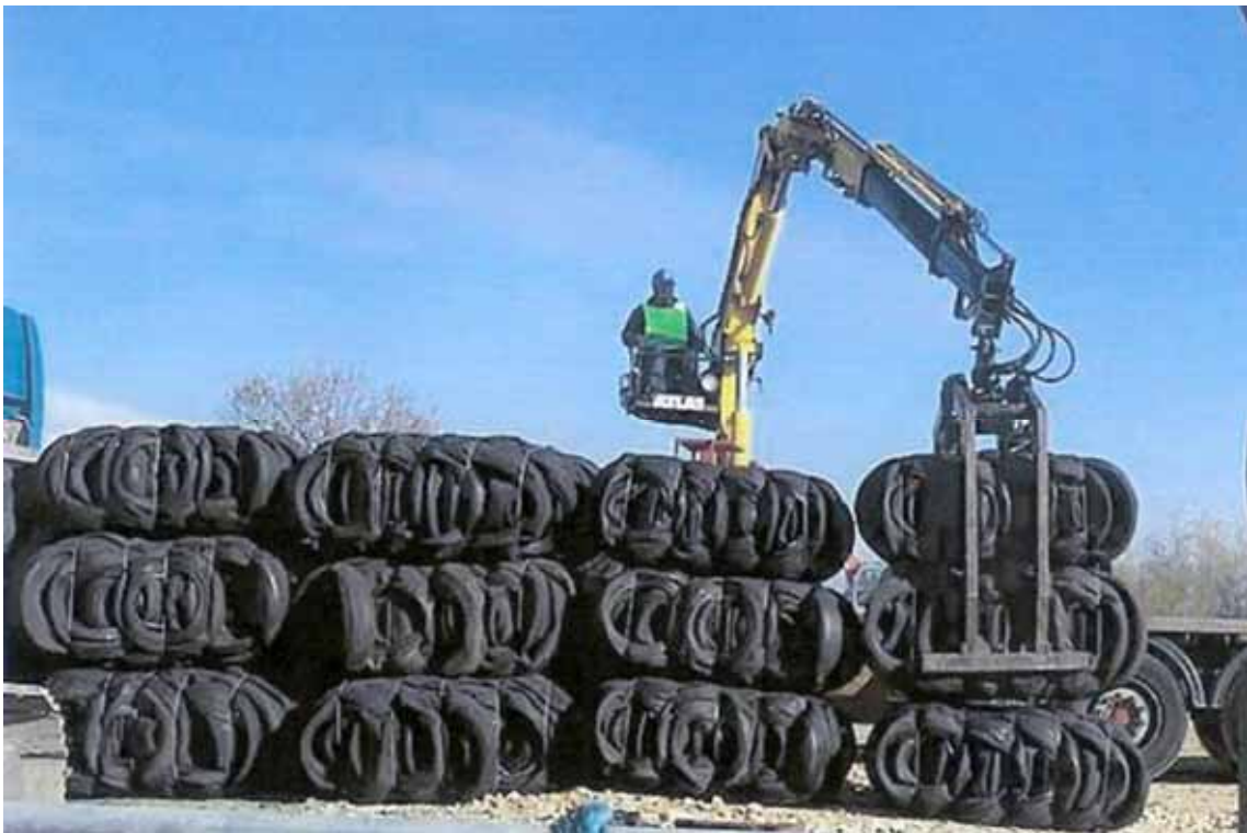
Figure 4.5 Offloading tyre bales from a delivery vehicle at a project site. (courtesy Environment Agency)
