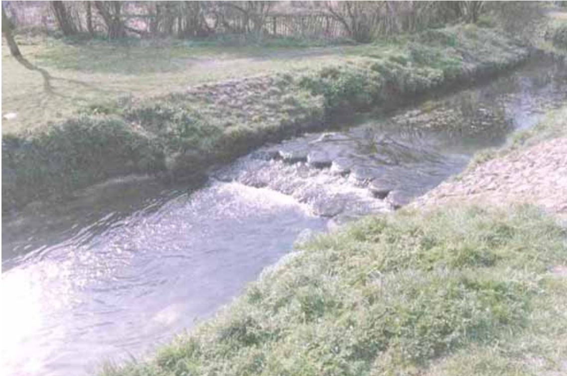
Figure 5.16 One of the tyre weirs in Limbury Park, Luton before removal (courtesy Environment Agency)
