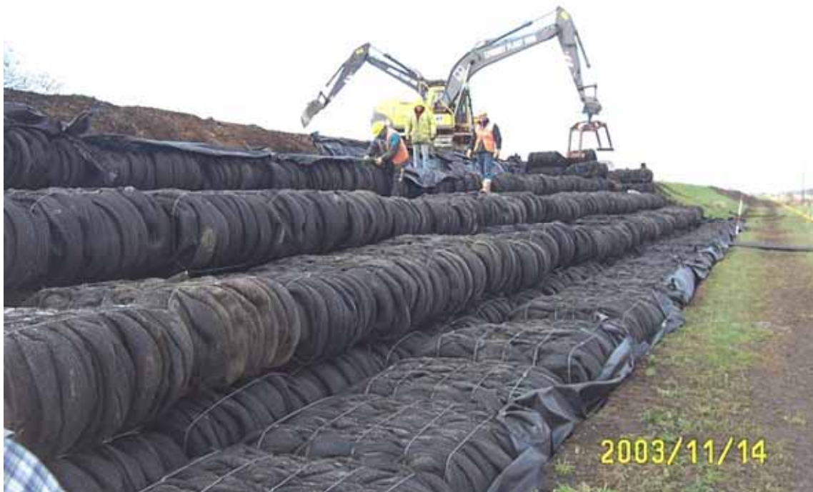
Figure 5.32 Construction of the River Witham Flood Embankment, near Lincoln (courtesy Environment Agency)
