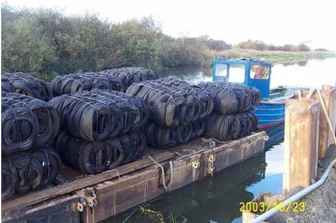
Figure 4.6 River transport of bales on final journey to construction site (courtesy Environment Agency)
