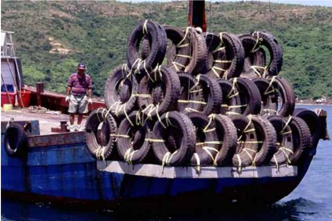
Figure 5.20a Open lattice reef structure (using either just 4, or 13 or more tyres held together by stainless steel bolts and with the basal tyres filled with concrete)
