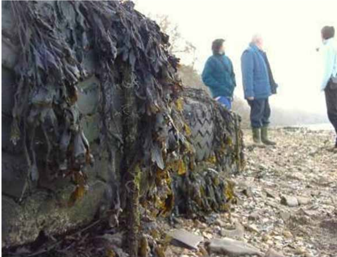
Figure 5.9 Algal growth on the Copperas Wood tyre embankment (courtesy Dr Ken Collins)
