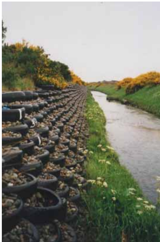
Figure 5.2 The tyre revetment beside the Mill Burn (courtesy Environment Agency)
