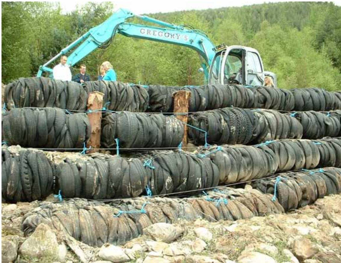
Figure 5.33 Construction of the Enrick embankment (courtesy Northern Tyre Recycling)
