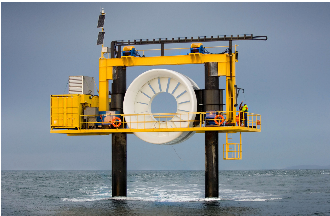
Figure 3-11: Installation of an open center current/tidal turbine.
