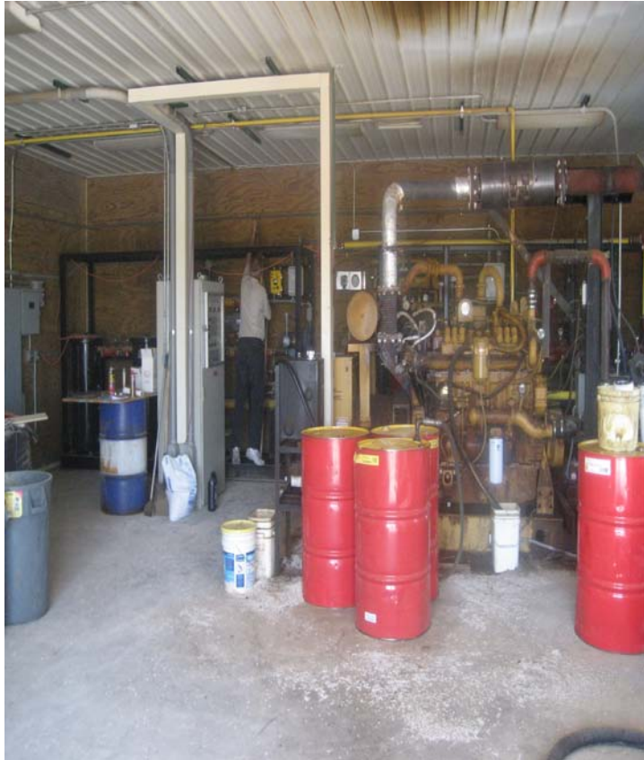
Photo 5.7.1 Electrical generator at Wyoming Premium Farms. Photo reflects the generator for AD Unit #2, an 80kWH unit installed in 2003. Generator is contained within a storage facility located next to the complete mix digester. Mr. Doug Derouchey, operations manager and minority owner, is adjusting the system controls in the left hand side of the screen
